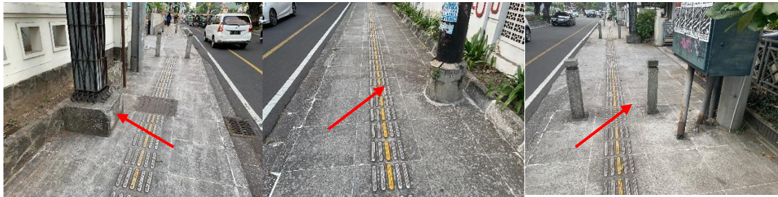
Figure 4. Road facilities such as electric poles that reduce the width of pedestrians
