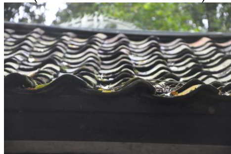
Figure 9. The roof covering uses tiles (Author Documentation)
