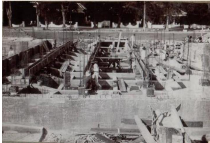
Figure. 1 The Construction process of the Balai kota Cirebon
