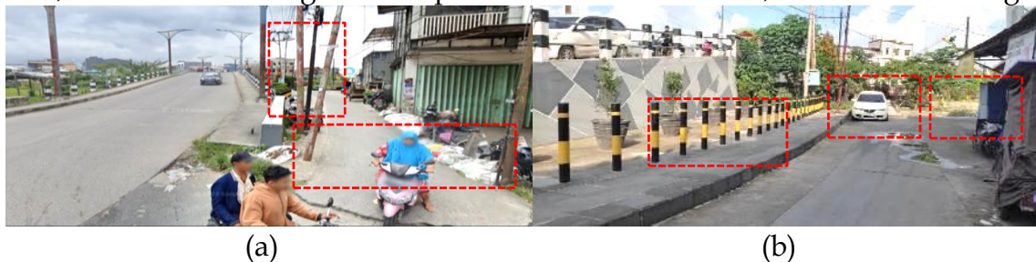
Figure 2. Western Entrance. (a) Objects Around Entrance, (b) Vehicle Circulation and Hard Material Elements
